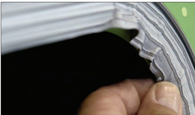
Figure 26: Wrapping the tape around a curve
